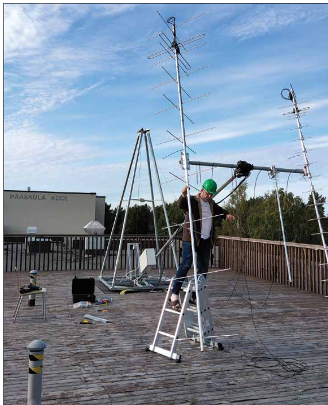
ES1TN SAT-side antennide paigaldamine
